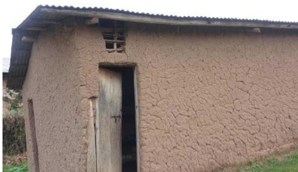
Figure 19: Store of Plates
