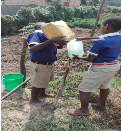
Figure 36: Newly constructed tippy tap with water and liquid soap for boys section
