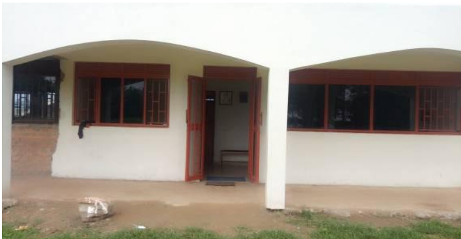
Figure 7: The main office/administration block.
