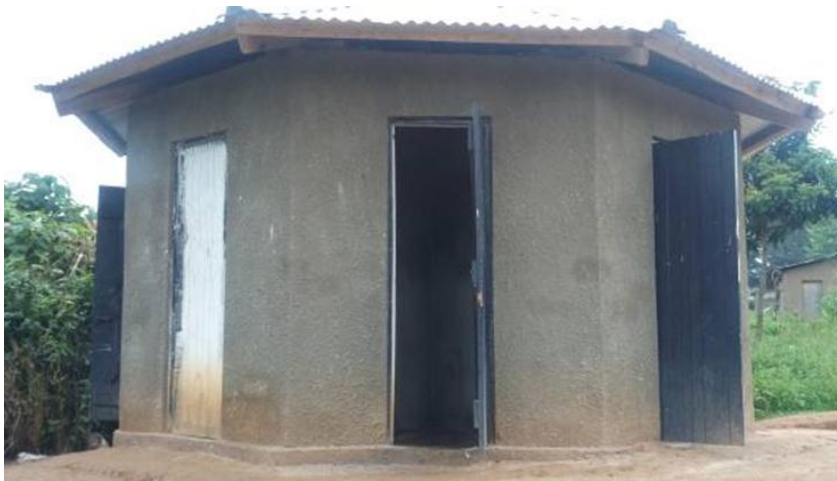
Figure 35: Picture showing a latrine which had no hand washing equipment
