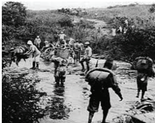
Figure 6.5: Lack of proper roads
